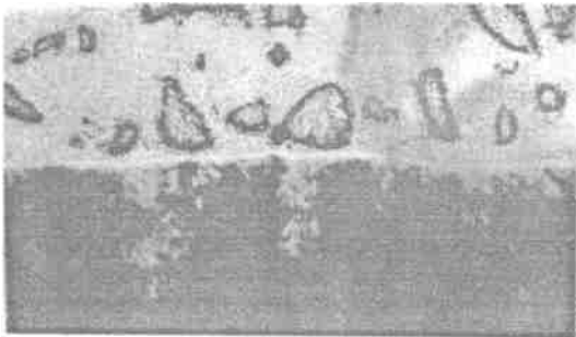
Fig. 2 Bonding interface between coating and substrate
